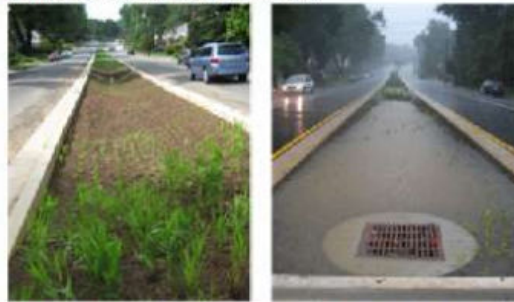
Figure 2. Constructed Green Street in Arlington County before (left) and during (right) a storm.
